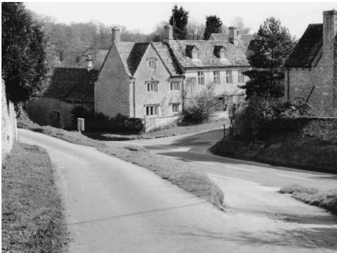
Arlington Manor viewed from the lane leading out from The Green. The mix of grassy banks and narrow lanes, seen in the foreground, are an important part of the character of this part of Bibury. Arlington Manor is of two dates and architectural styles, the gabled part dating from the mid-seventeenth century, and the larger formal part to the right being of about 1720.
