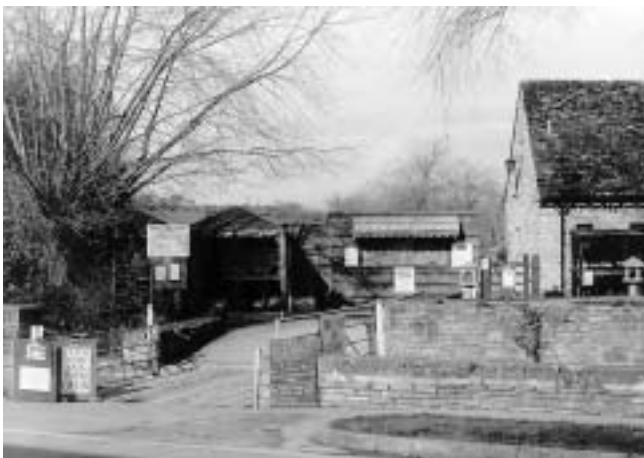
Sales kiosks and signs around the well-designed main trout farm building spoil this otherwise attractive part of the conservation area.
