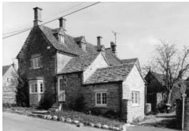
The recent extension to this listed building in Arlington has been sympathetically designed with appropriate local materials. Officers of the Council gave advice that led to this successful solution.
