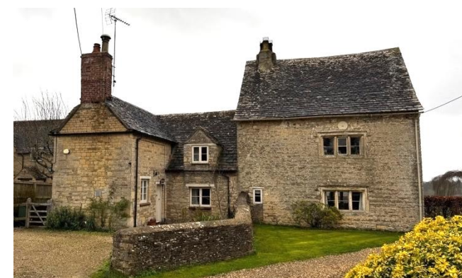
Fig 7.1.3.1 Nos. 37 and 38 (Grade II): likely former farmhouse with several former barns and other former agricultural buildings in the vicinity.
