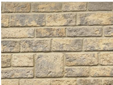
Fig 7.4.1.1 (above top) Coursed local rubblestone
