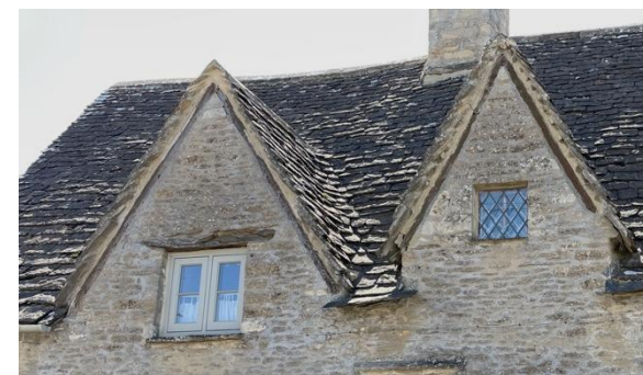
Fig 7.4.2.1 (top left) Diminishing courses of stone tiles swept to valleys.
