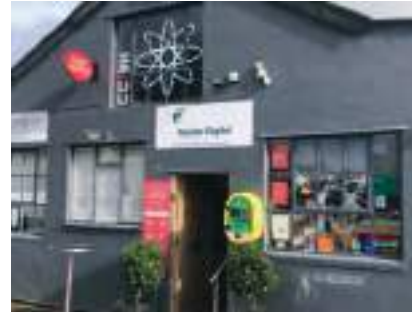
Post Office Defibrillator 2c The Cambrook, High Street, Chipping Campden, GL55 6AT
