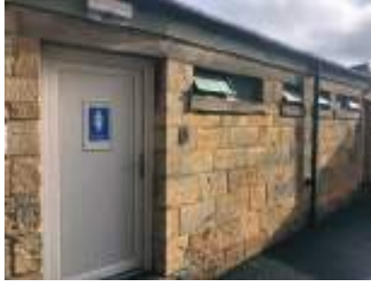
Toilets at Visitor Information Centre The Old Police Station, High Street, GL55 6HB
