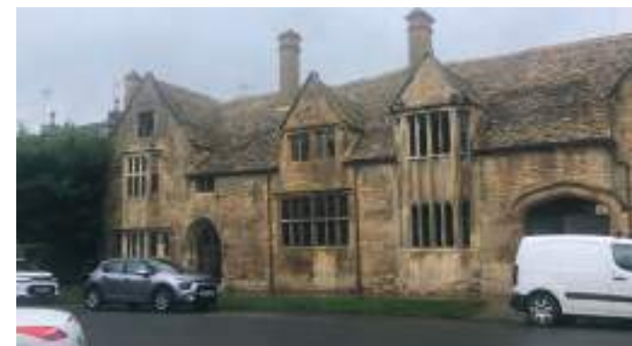
Figure 12: Grevel House; 14th Century, Grade I listed.
