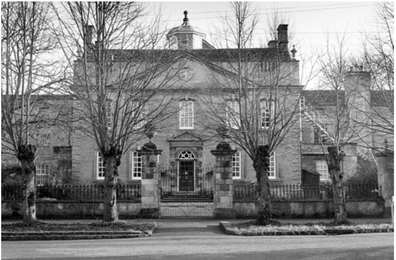
The fine palladian facade of Harrington House can be seen behind low walls, topped with spearhead railings and linked to rusticated gatepiers, all of which contributes greatly to the character of the conservation area and deserve careful consideration.
