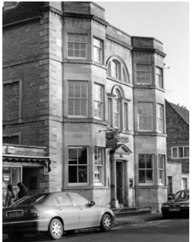
Lloyds Bank occupies a grand, late 18th Century former house. This displays classical features of that date, including diocletian windows, a pedimented doorcase, rusticated quoins and full-height canted bay windows.
