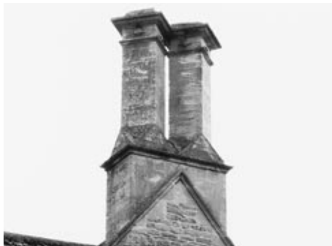
Several buildings in Bourton have diagonally set chimney stacks, occasionally rising laterally from the side walls, as seen here at Riverside House.
