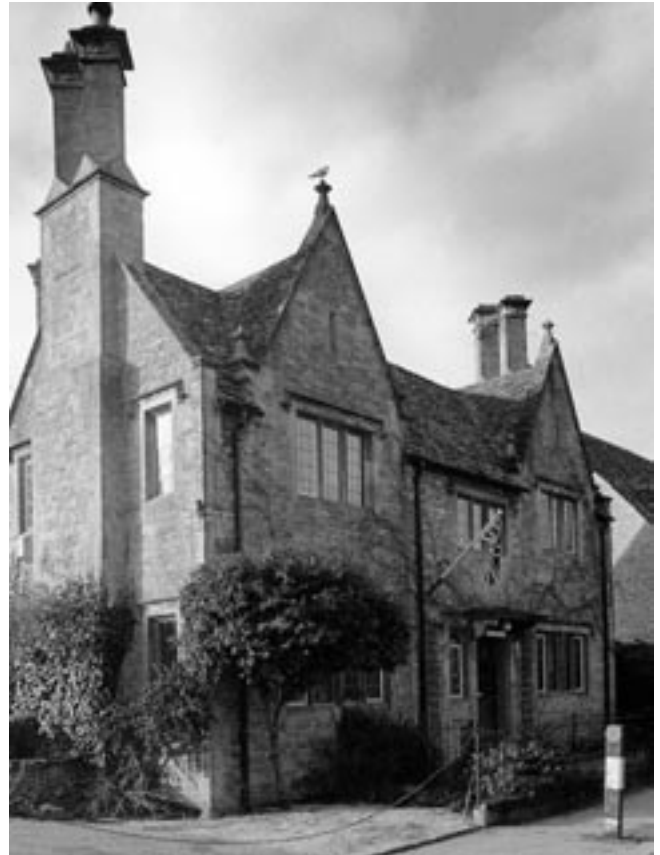
The Cotswold Tudor Revival style house 'Fairlie' is set back from the river and is characterised by steep gables topped by finials and paired diagonal chimneys.
