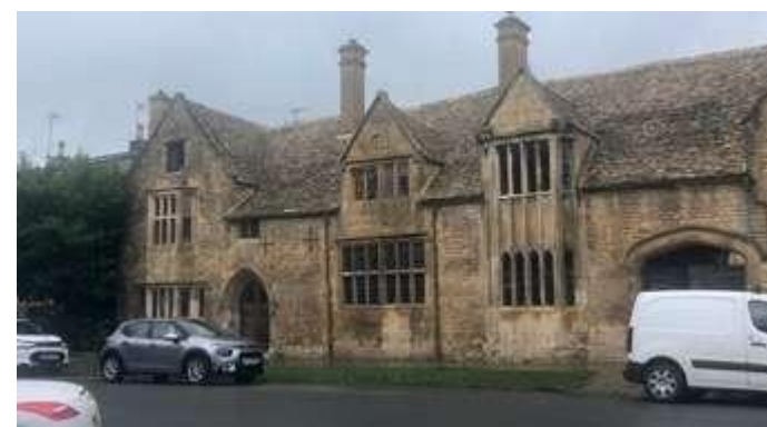
Figure 12: Grevel House; 14th Century, Grade I listed.
