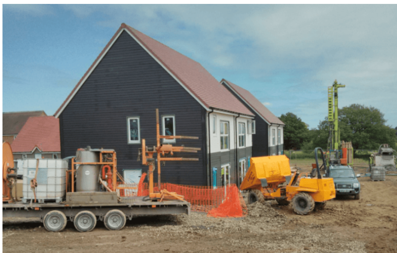
Figure 7 Installation of a shared ground loop array for ground source heat pumps in new build social housing
