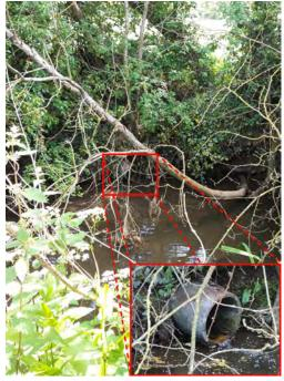
Photograph 13 – Highway drain outfall into Poulton Brook
