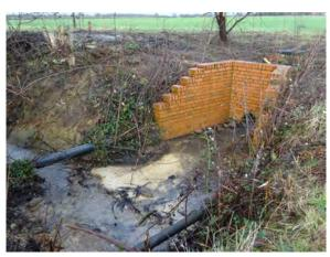
Photograph 8 – Headwall from Pipe C into Drain C (January 2024)
