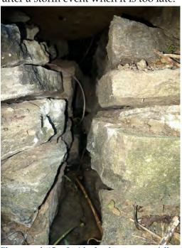
Photograph 15 – Inside the dry-stone outfall from Pipe B
