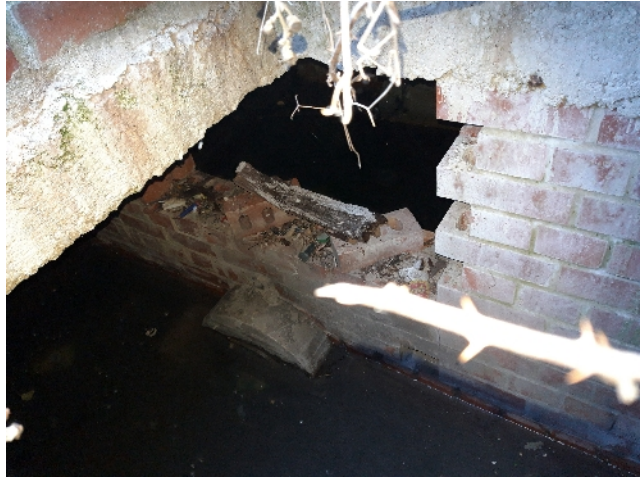
Photograph 5a - Inside the manhole
