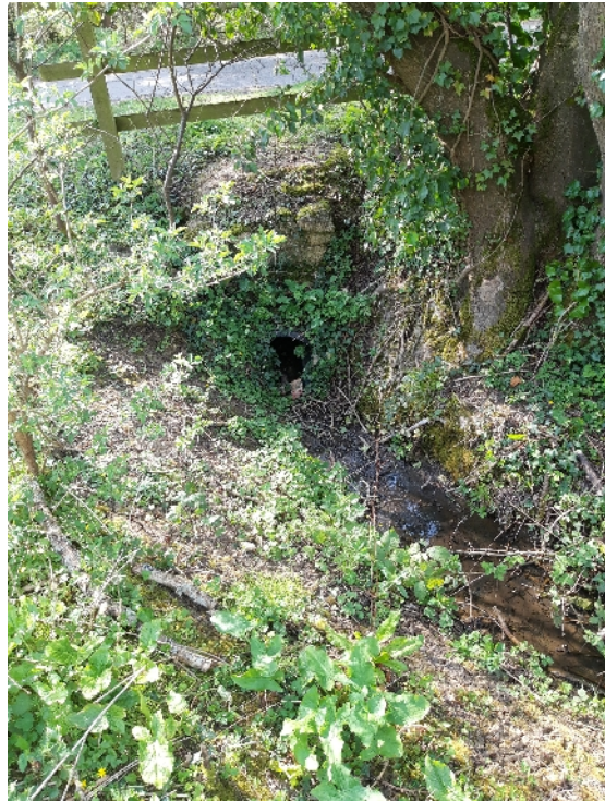
Photograph 7 - Drain E Looking back to Oak Road
