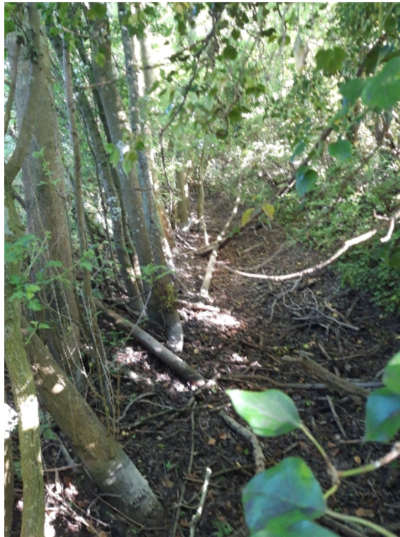
Photograph 6 - Drain C looking South
