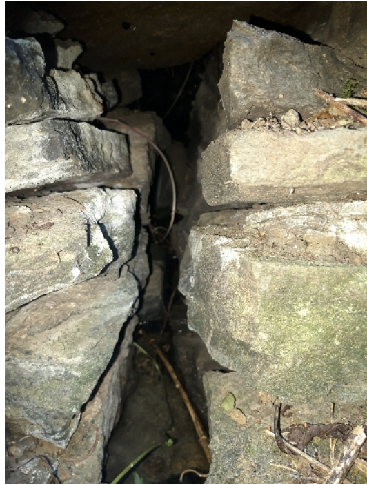
Photograph 12 - Inside the dry-stone outfall
