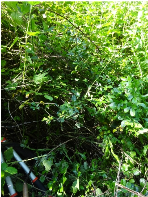
Photograph 8 - The point where the 9” pipe joins Drain E
