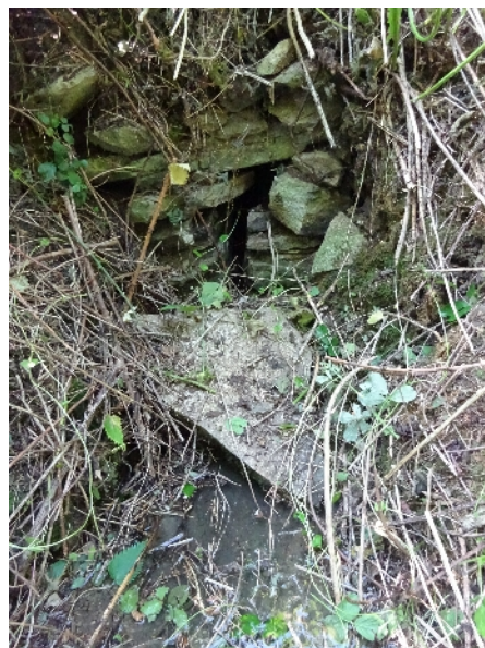
Photograph 9 - The headwall of the pipe joining Drain E after clearing
