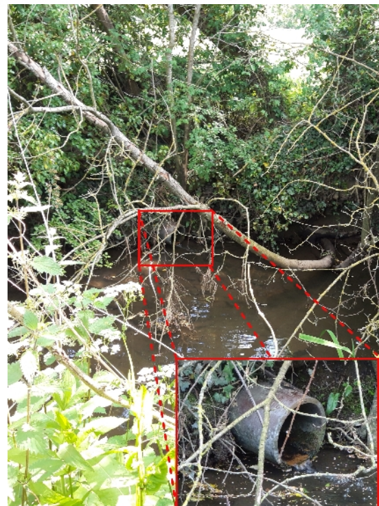
Photograph 10 – Highway drain outfall into Poulton Brook
